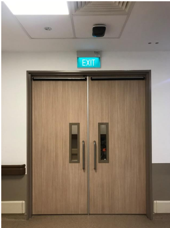
Fig. 2 Photograph shows real-time location system detector installed at the ceiling of the entry and exit points of different areas in the emergency department.
